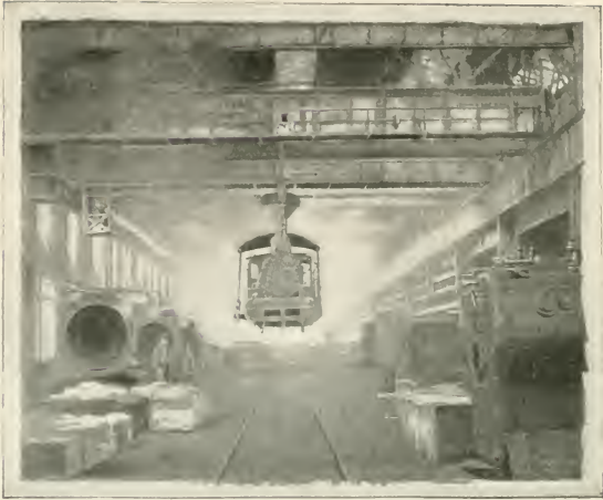
An American Electric Travelling Crane, Nijni Novgorod, Russia.
